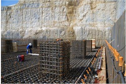
Sitting atop the lower basemat, 500 of these 1.8 metre concrete columns will support the seismic pads. These, in turn, will support the upper basemat of the Tokamak Complex—the actual "floor" of the installation (August 2011).
