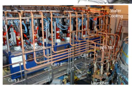
Total 3MW high power klystrons for LHCD. Additional klystrons have been purchased to raise the power to 4MW
