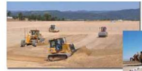
Bulldozers and scrapers are busy leveling the 14,000 square-meter area that will host the huge PF Coils Assembly Building.
