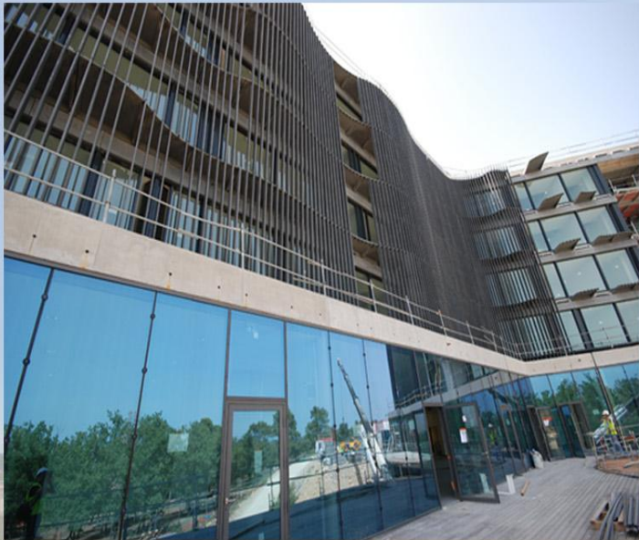
Staff will move in to the ITER Headquarters building this fall. Photo: ITER Organization
