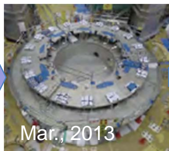
Cryostat Base (260 tons)
