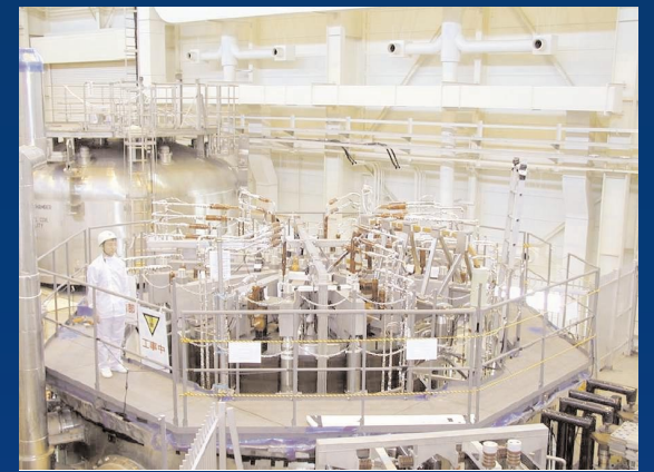
Model coil and insert coil installed at the test facility in JAERI Naka. In the background is the vacuum chamber lid.
