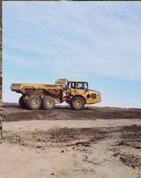
Initial Site Road Construction - Complete
