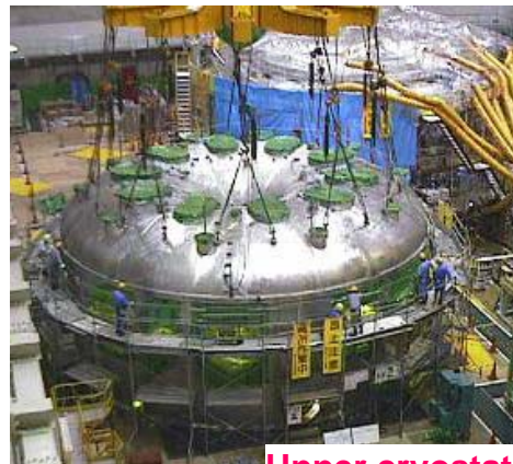
Upper cryostat
