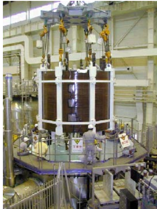
Figure 5.2-1 CS Model coil. The Outer Module being placed outside the Inner Module which has already been installed in the vacuum chamber.
