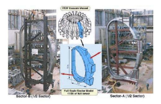
Figure 3.6 Full scale ITER Vacuum Vessel sector prototype constructed in Japan. Courtesy of ITER.
