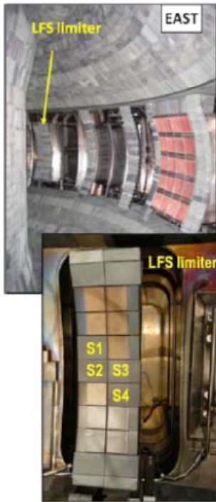
Figure 1. Interior of EAST (top) with location of startup-limiter; closeup of limiter (bottom) with coated tiles (S1 ... S4) indicated.
