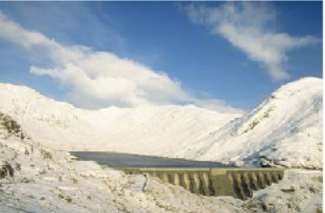
Pumped storage - 30 Cruachans (30b) Upgrade Anglo-Scottish interconnector (1b)
