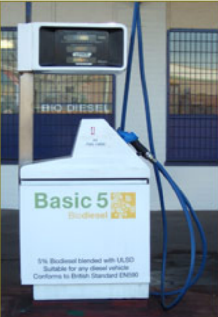
A pump full of B5
