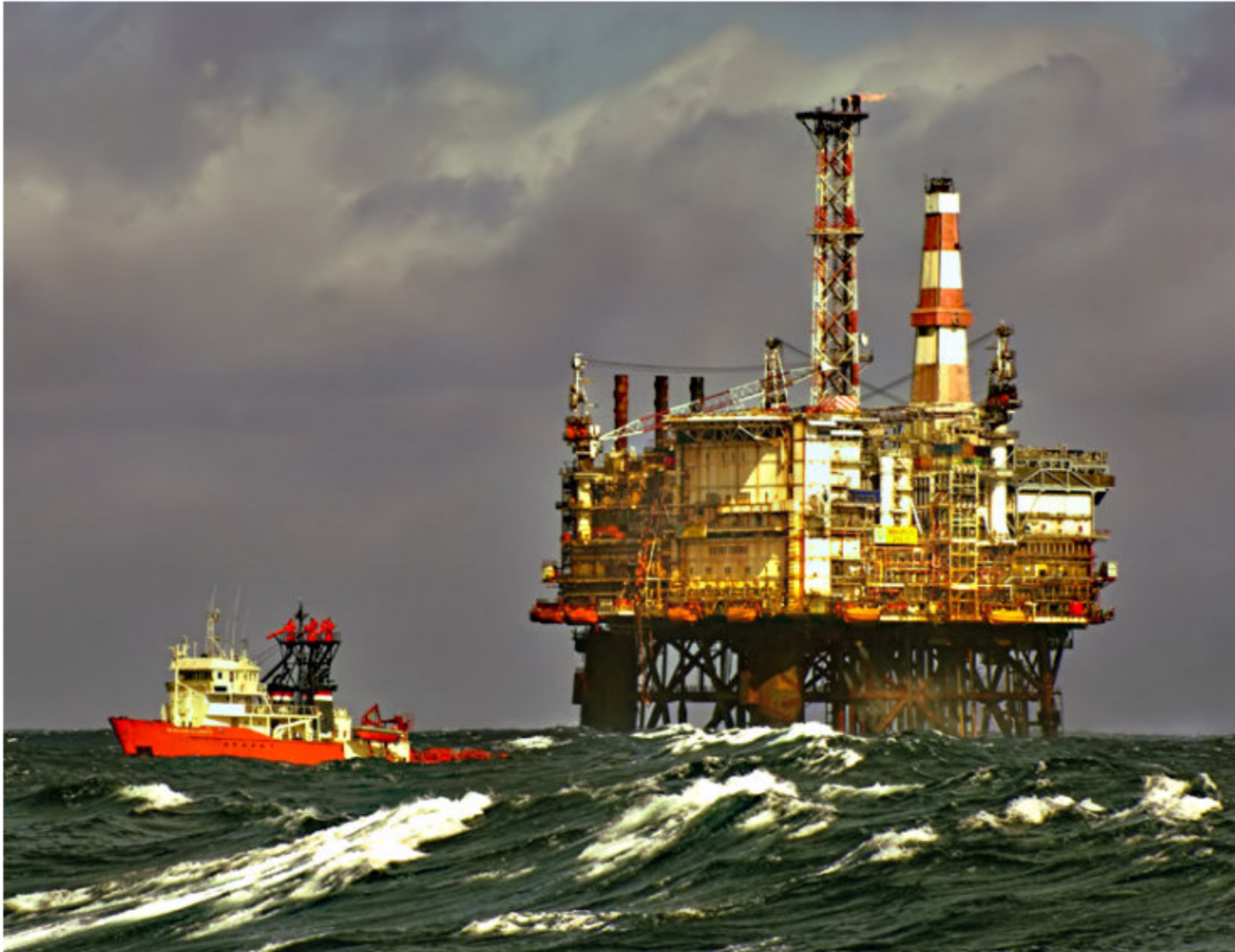
Magnus platform - delivers 5GW; 71,000 tonnes of steel
