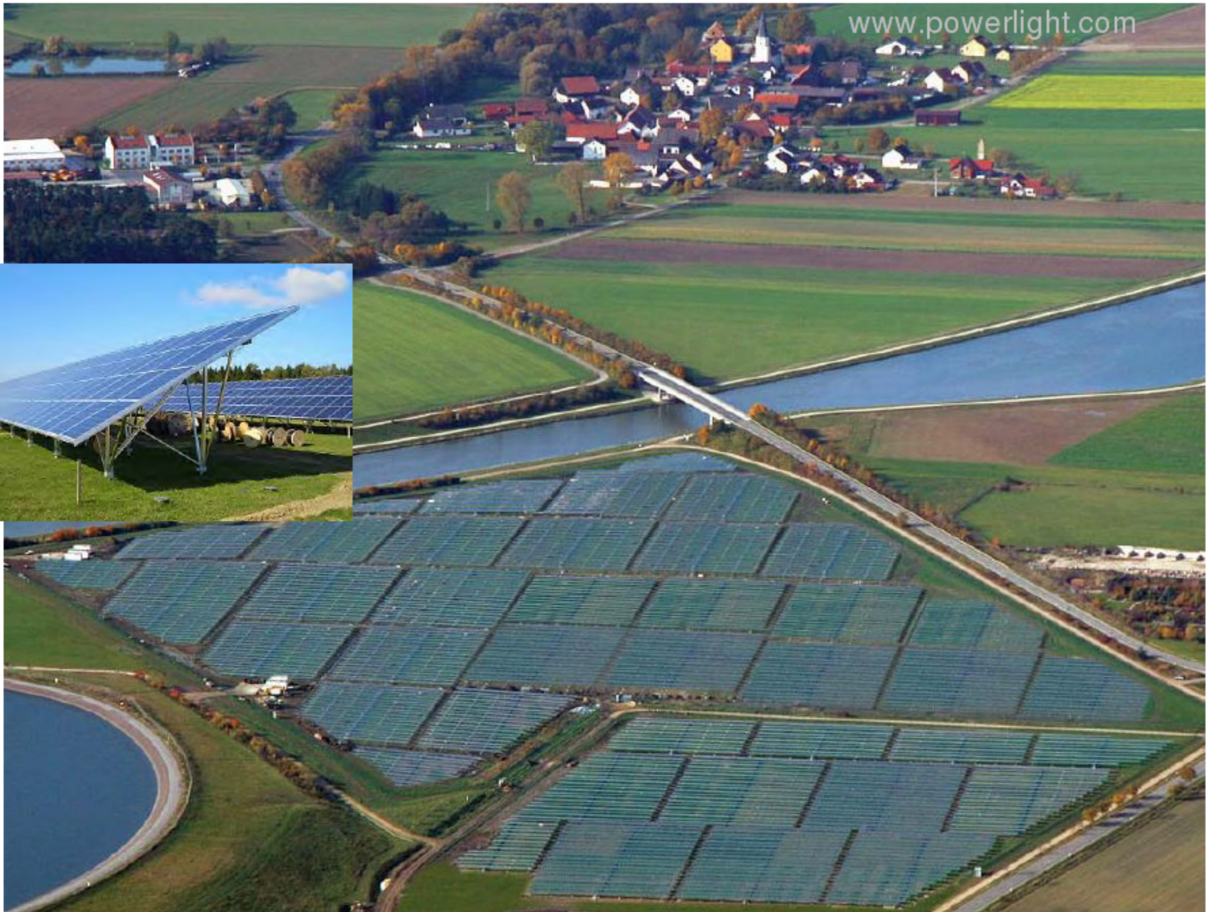
Bavaria Solar Park: 5 \text{ W/m}^2 ; this picture shows 0.7 \text{ MW} (average)
