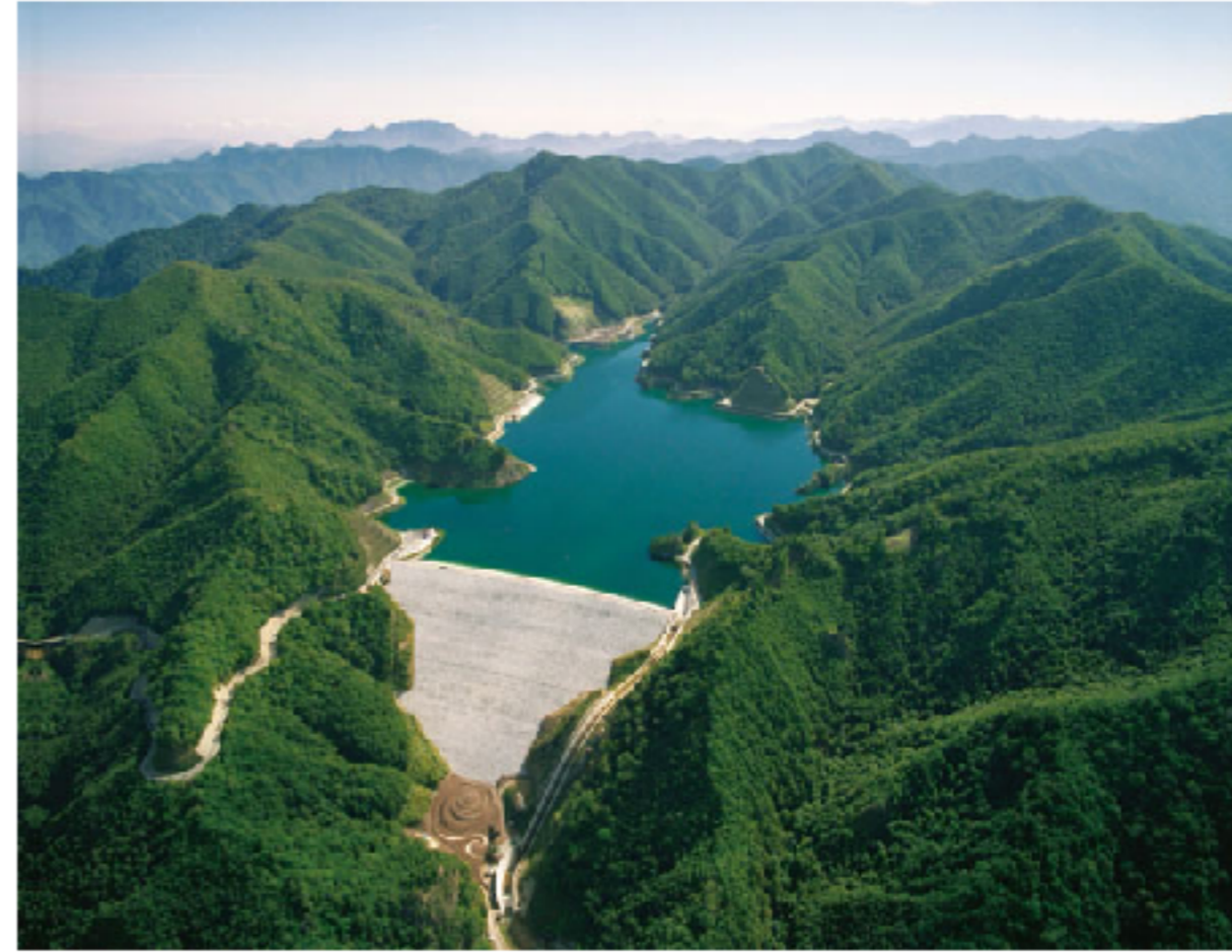
Kannagawa Power Plant (29 GWh)
