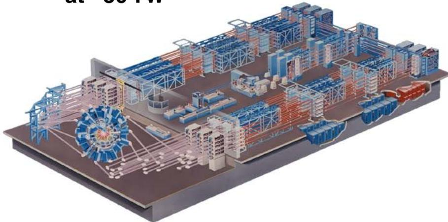
**The OMEGA EP laser delivers ~2-kJ IR light in 10 ps (~2 PW) and 20-kJ light in UV-ns pulses**
