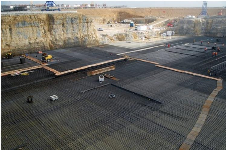
Steel reinforcement bars—each one weighing nearly 100 kilos—are built up to 1.5 meters on the floor of the Seismic Pit. In the distance, the future ITER Headquarters buildings rises above the platform. (August 2011).
