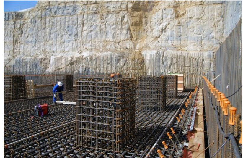
Sitting atop the lower basemat, 500 of these 1.8 metre concrete columns will support the seismic pads. These, in turn, will support the upper basemat of the Tokamak Complex—the actual "floor" of the installation (August 2011).
