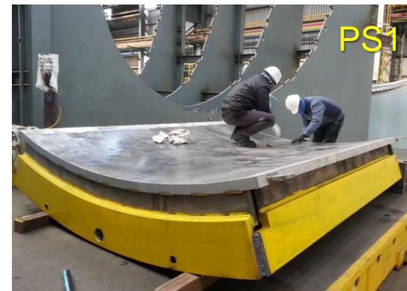
◀ Completion of inner and outer jigs for welding after forming of inner shell of inboard segment (PS1)
