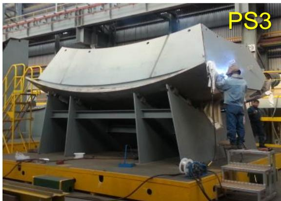
◀ Start welding after inner and outer jigs for inner shell of equatorial segment (PS3)
