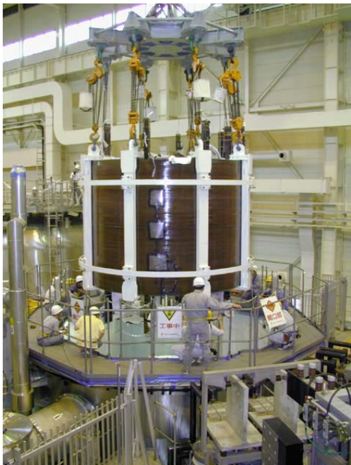
FIG. 5: Central Solenoid Model Coil Facility
