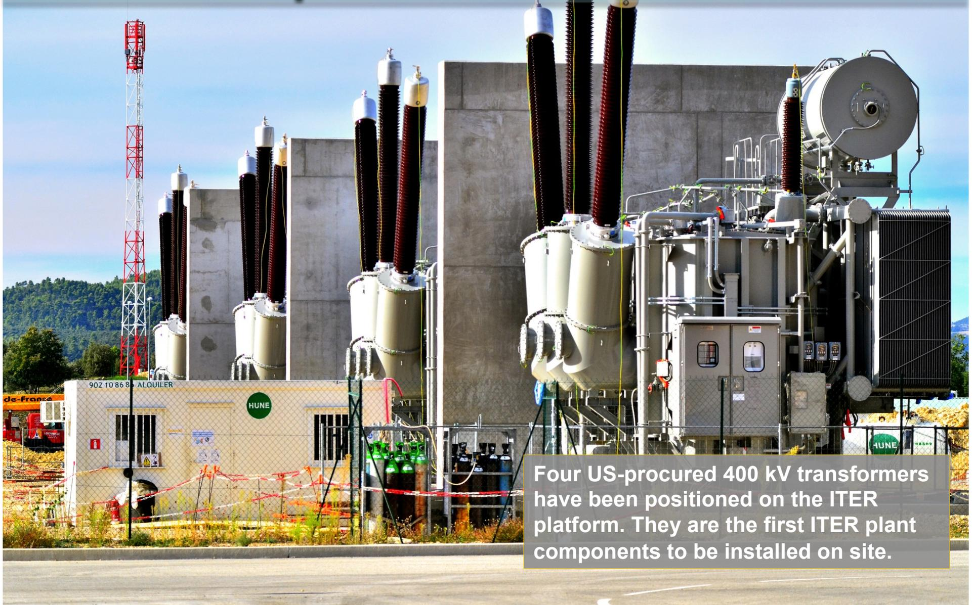
Four US-procured 400 kV transformers have been positioned on the ITER platform. They are the first ITER plant components to be installed on site.
