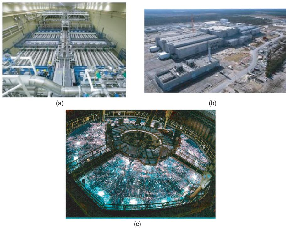
**Figure 3.** (a) The NIF main amplifier laser bay which was completed and achieved an output energy of 1 MJ. (b) The laser and target chamber buildings of LMJ at CESTA/CEA, Bordeaux, France, which will be completed in 2014. (c) The Z-Machine: a pulse power machine to produce a high power x-ray of megajoules.
