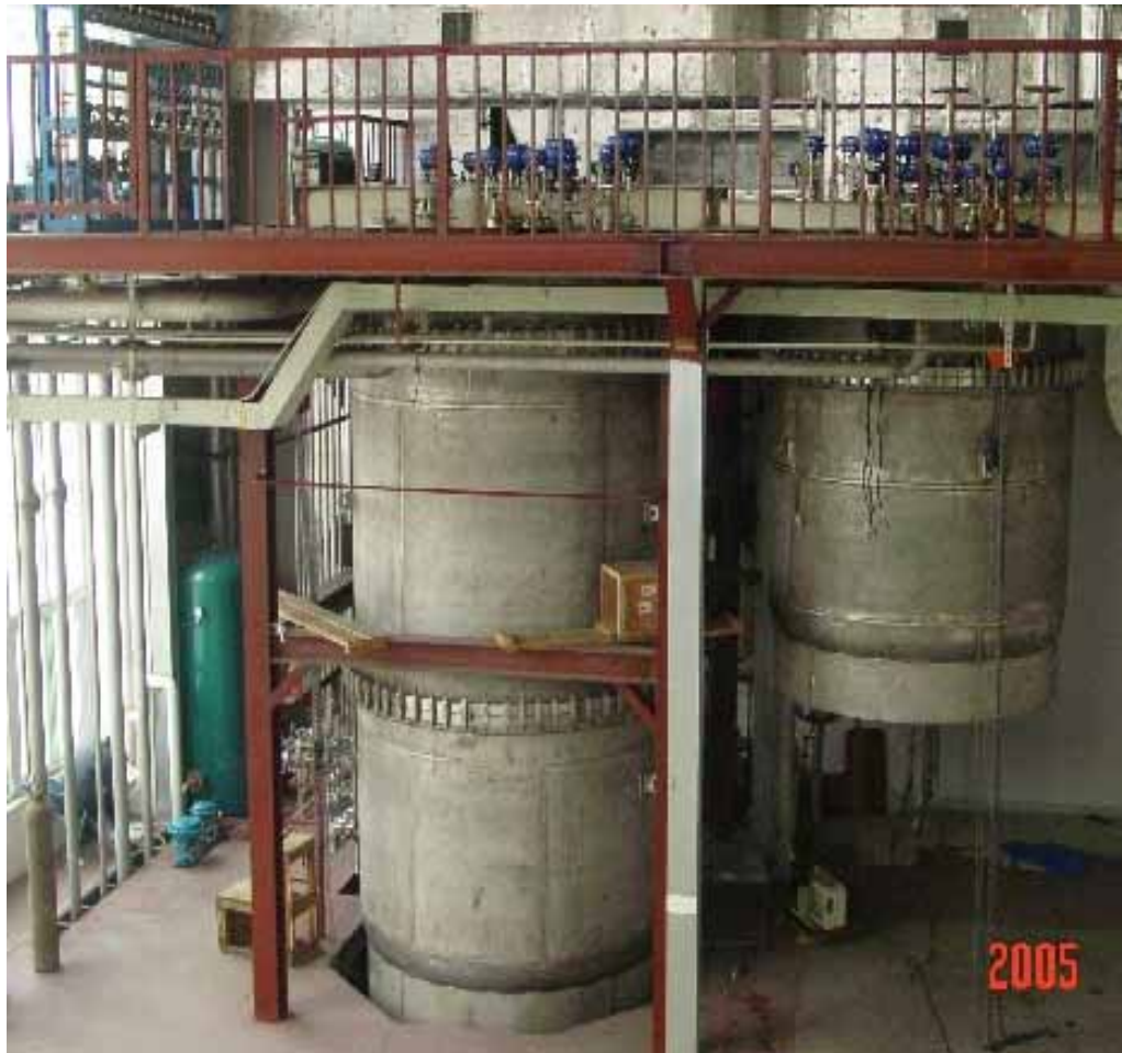
2kW/4.4K+11kW/80K refrigerator
